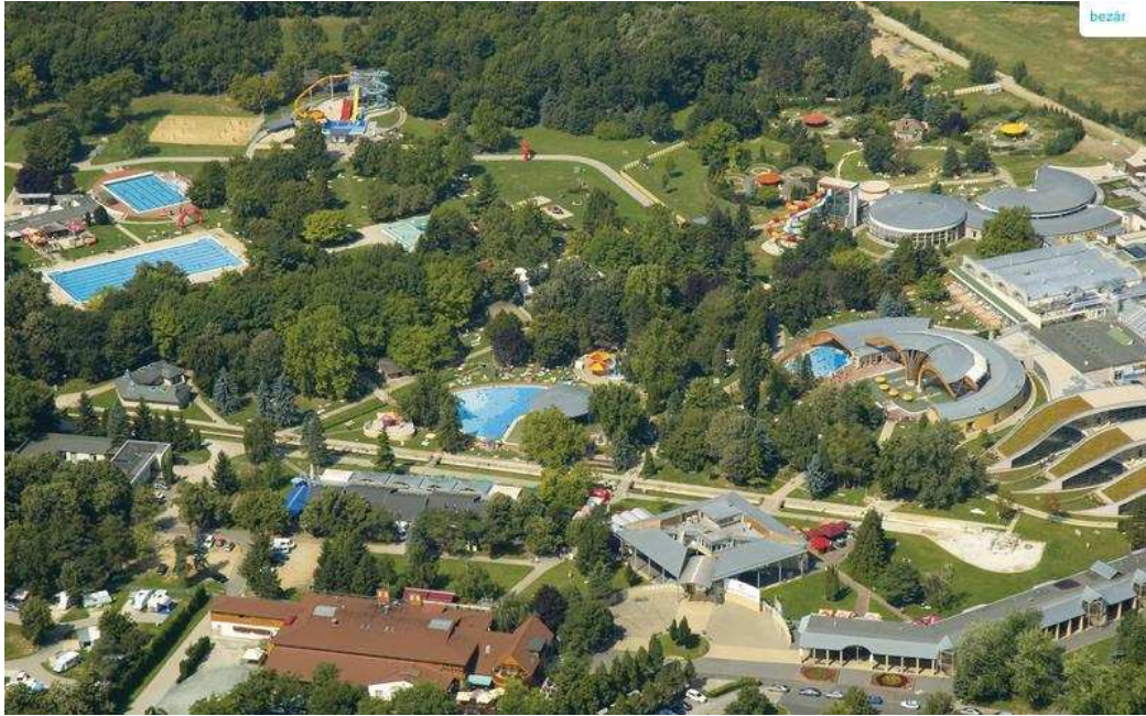
Figure 26: Thermal spa at Bükfürdő
